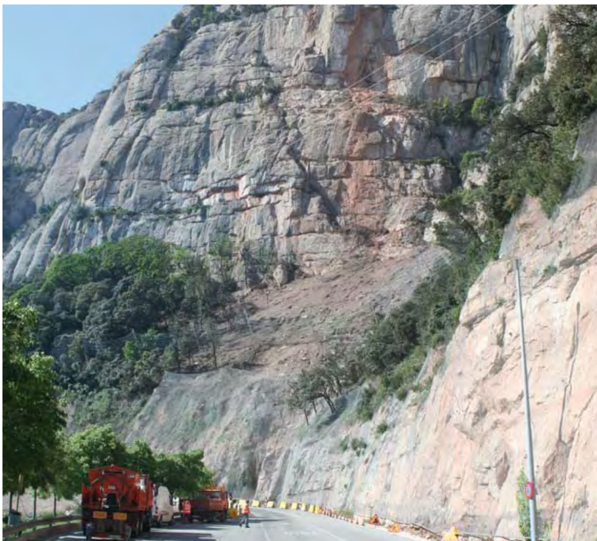
51 The large rock landslide in January 2007 in Montserrat (Photo IGC).
