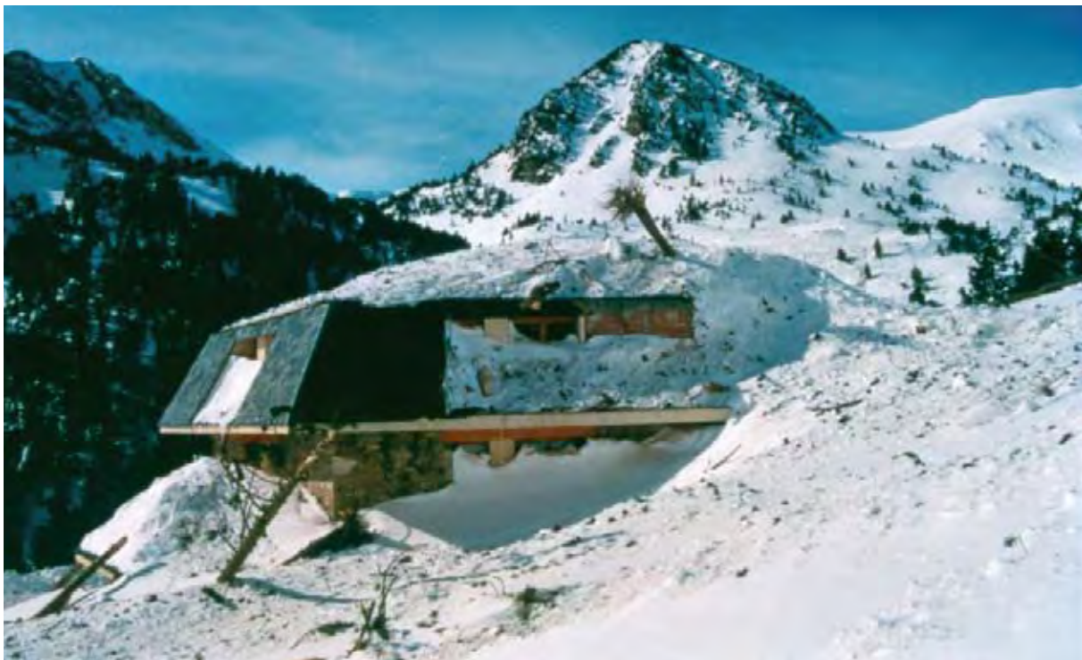
Impact of an avalanche on a building during the episode of February 1996 in the high Ter valley. (Photo Hostal Pastuira courtesy of the I'IGC).
